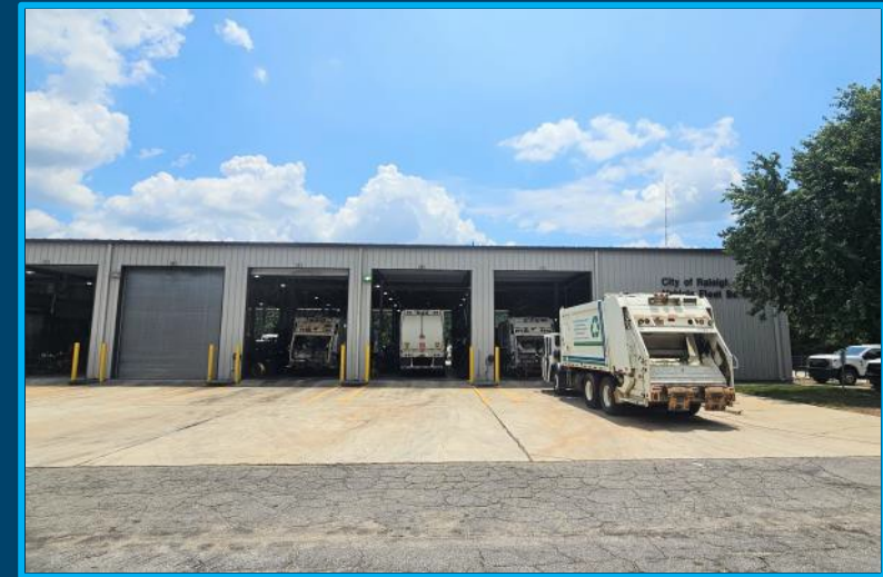
Heavy Equipment Shop
