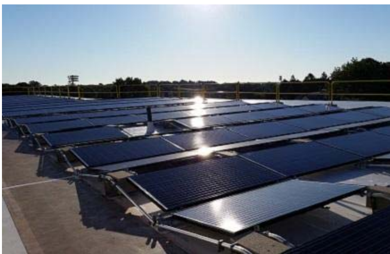
Figure 13: Example of East-West Racking by Zep Solar (Photo courtesy of Zep Solar)
