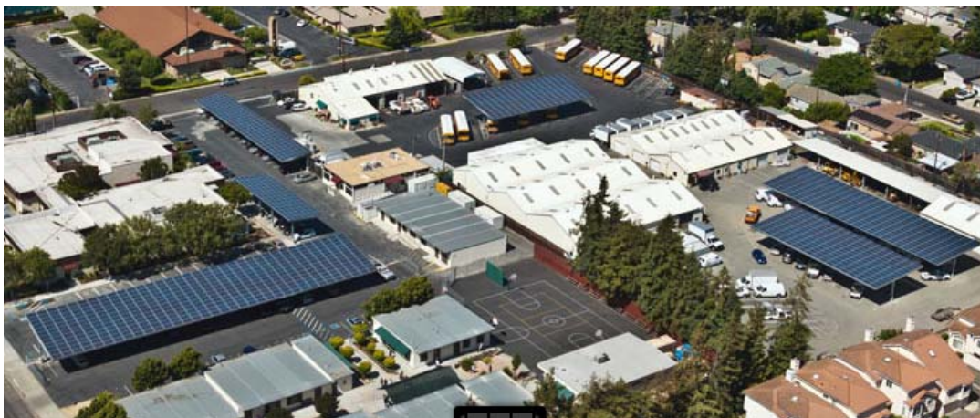
Figure 3: Example Parking Lot PV Shade Structures at a School in the Santa Clara Unified School District in California (Photo: Borrego Solar)
