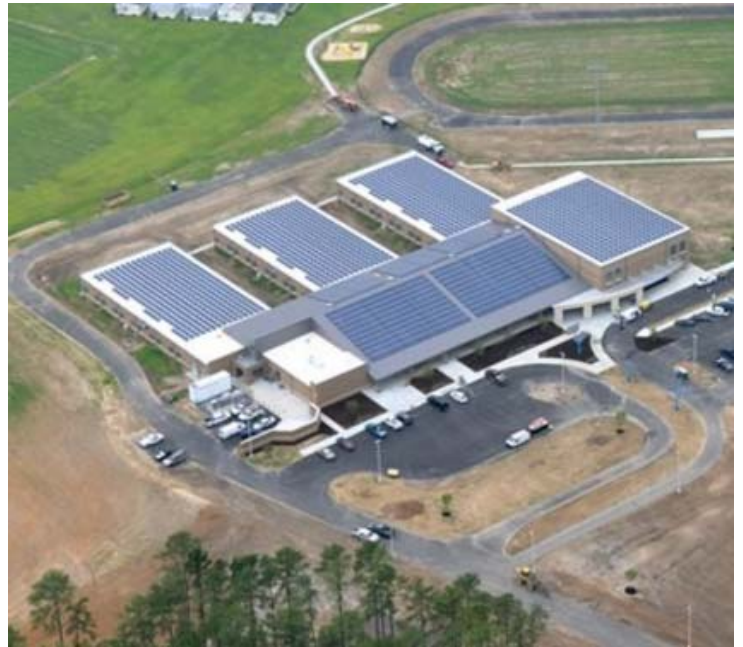
Figure 2: Solar PV on the Roof of Sandy Grove Elementary, in Lumber Bridge, NC (Photo: Sfl+a Architects)
